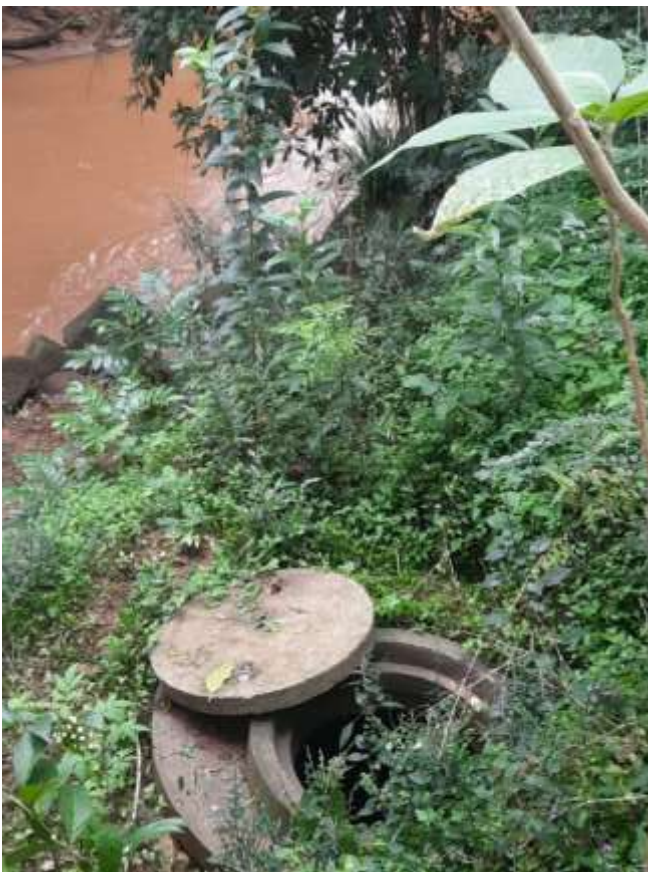
Plate 2: Existing stormwater manhole to be replaced
