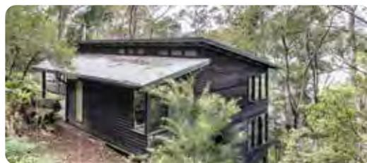
*Example of an unmaintained APZ. The house is surrounded by thick vegetation and the roof and subfloor areas could ignite in an ember attack.*
