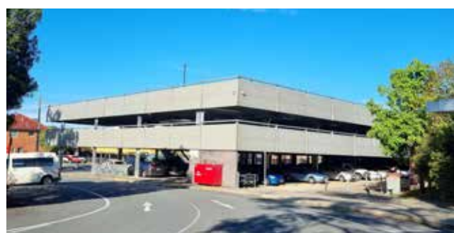
Murwillumbah multi-storey car park repairs now underway.
