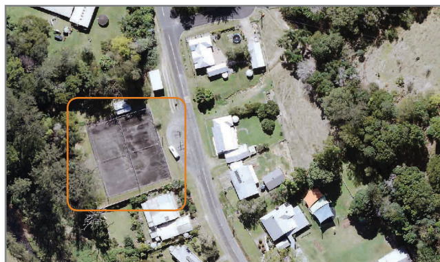
Chillingham tennis courts (highlighted) to get a makeover.
