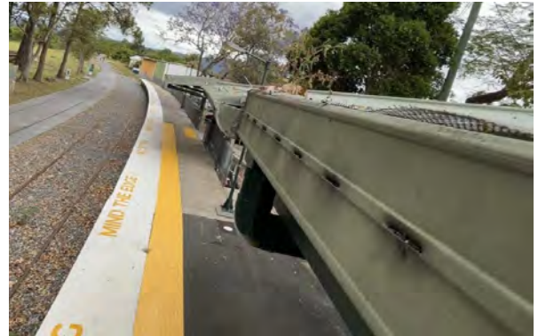
Picture 9 Platform awning with two gutter profiles
