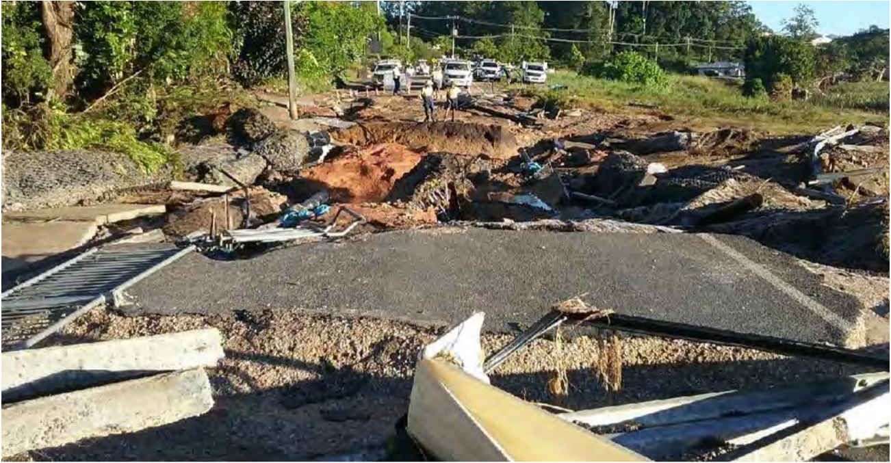
Blacks Drain located in South Murwillumbah was severely damaged by the 2022 flood. Council will be asking for tenders from contractors interested in completing the reconstruction works.
