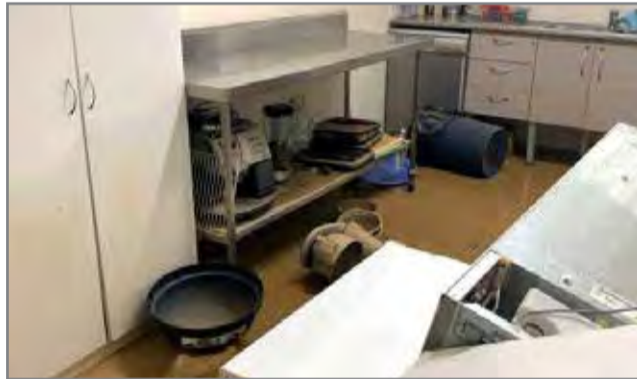
Murwillumbah Community Centre after the 2022 flood.
