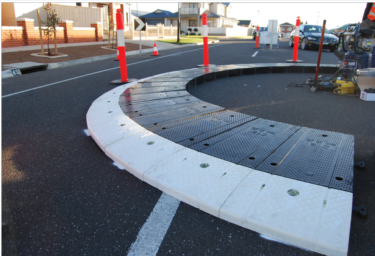
The Tweed's first rubber roundabout will soon be installed at Bilambil Heights, saving money and time compared to traditional methods.
