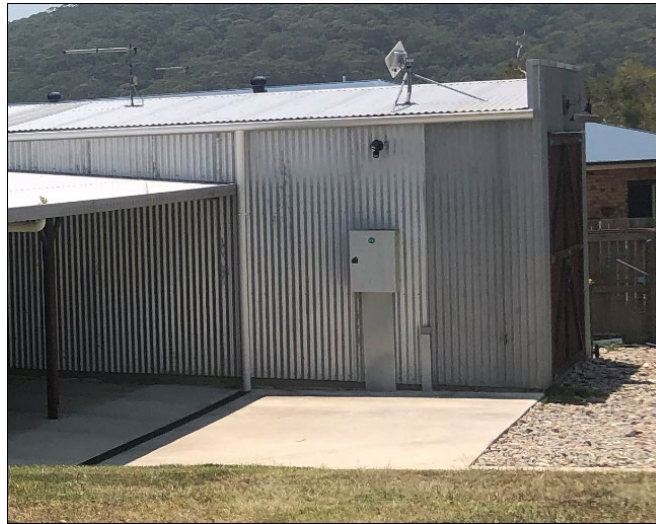
Figure 2 Example of weathered/dull zincalume cladding on the secondary dwelling (southern elevation)
