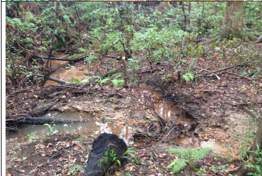
Pic 7 – Upstream section, channel scoured back to natural levels.
