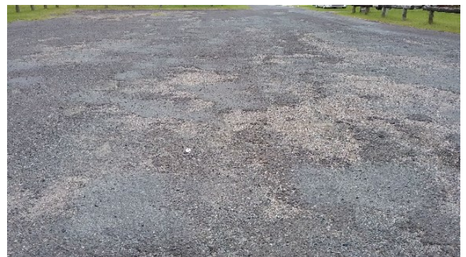
Aged surface condition if bitumen is not treated. Further deterioration will result in potholes and failures.
