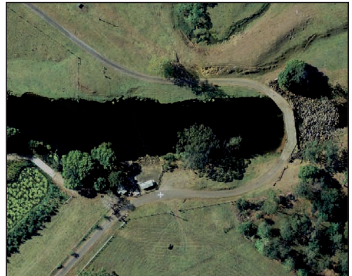
The existing Tyalgum Water Treatment Plant and weir.
