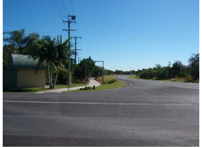
Photo 2: Tweed Coast Road – New recycled main to be installed for 430m along the western side of Tweed Coast Road between the road verge and footpath. The recycled water booster pump will be constructed adjacent to the rising main 35m from the connection point at the corner of Tweed Coast and Round Mountain Roads
