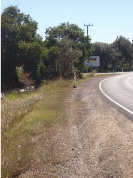
Photo 3: Tweed Coast Road – New recycled main to be installed for 430m along the western side of Tweed Coast Road between the road verge and footpath
