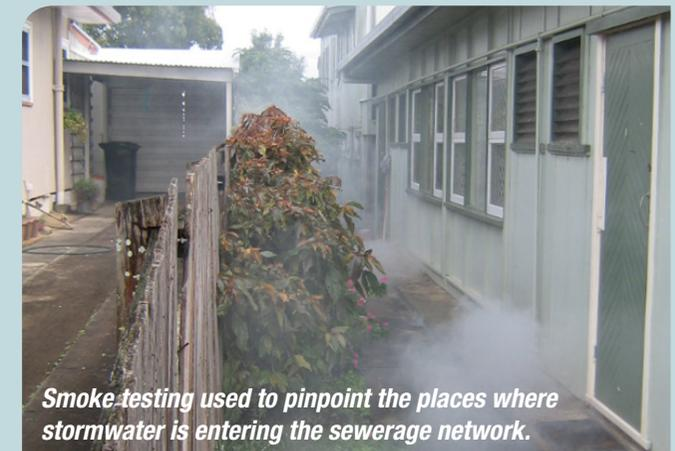
*Smoke testing used to pinpoint the places where stormwater is entering the sewerage network.*
