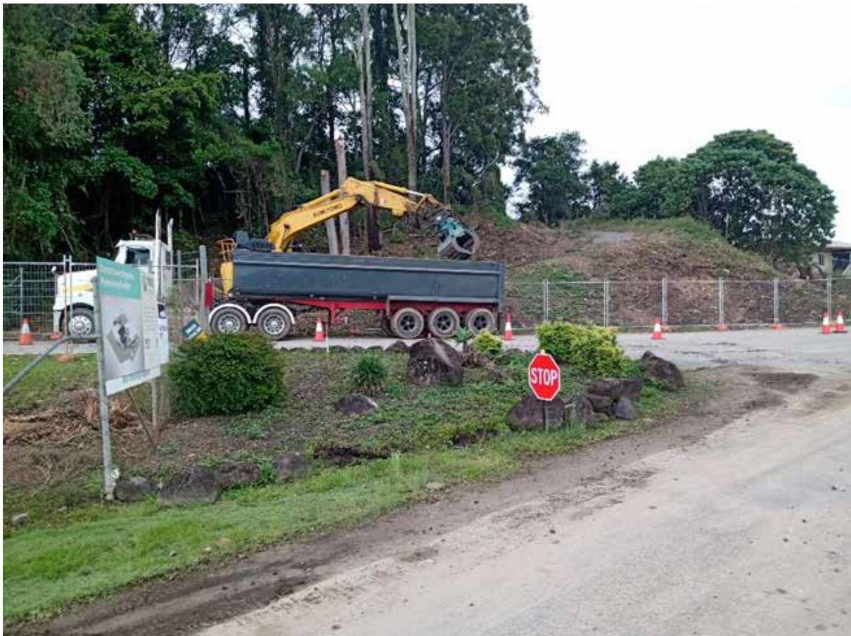
Work starting on the masterplan at the Stots Creek Resource Recovery Centre.
