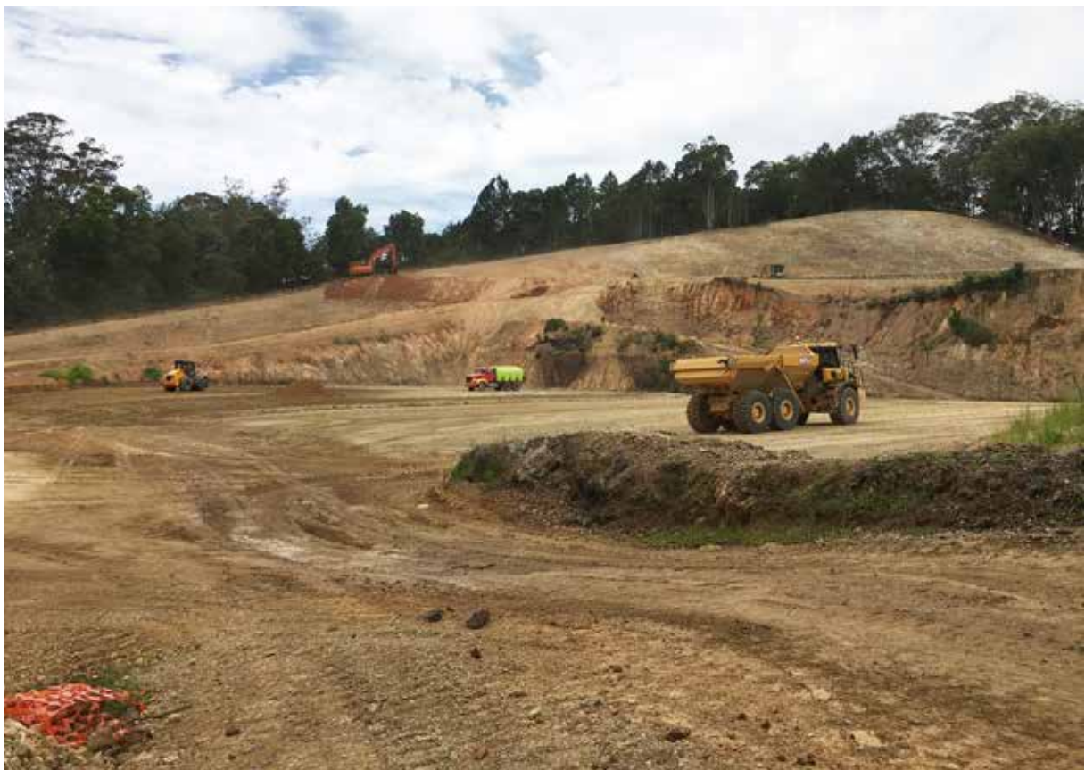
The Stotts Creek Resource Recovery Centre final landfill cell.
