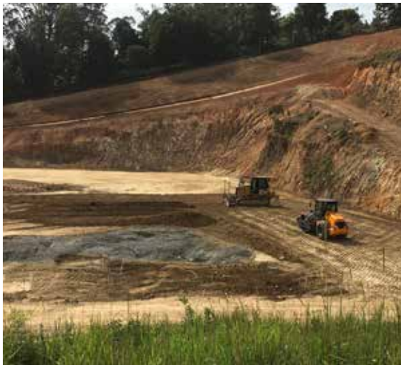
New landfill cell at Stotts Resource Recovery Centre.
