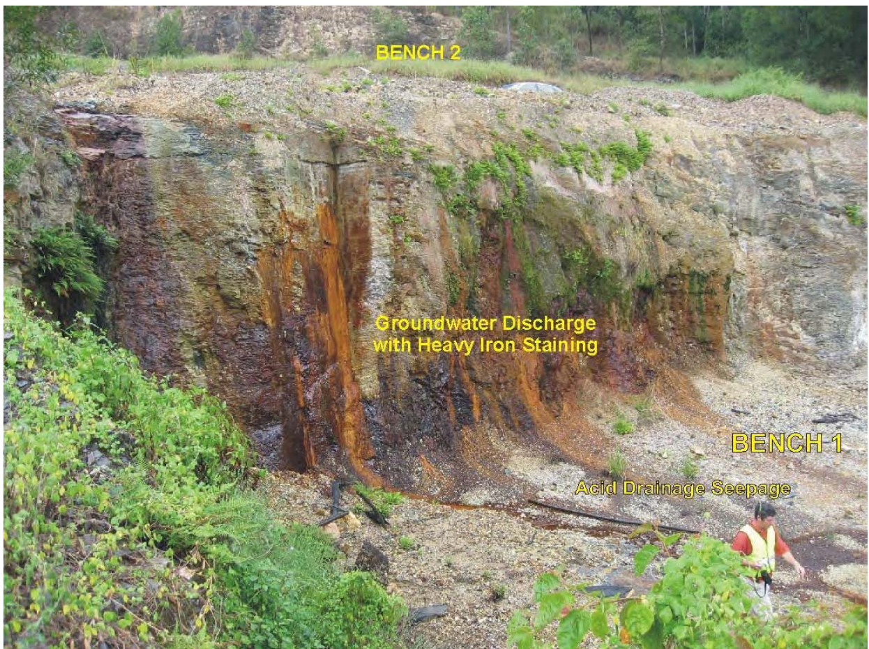
Face 1/2 Staining (Photo 8118 – 18/5/09)
