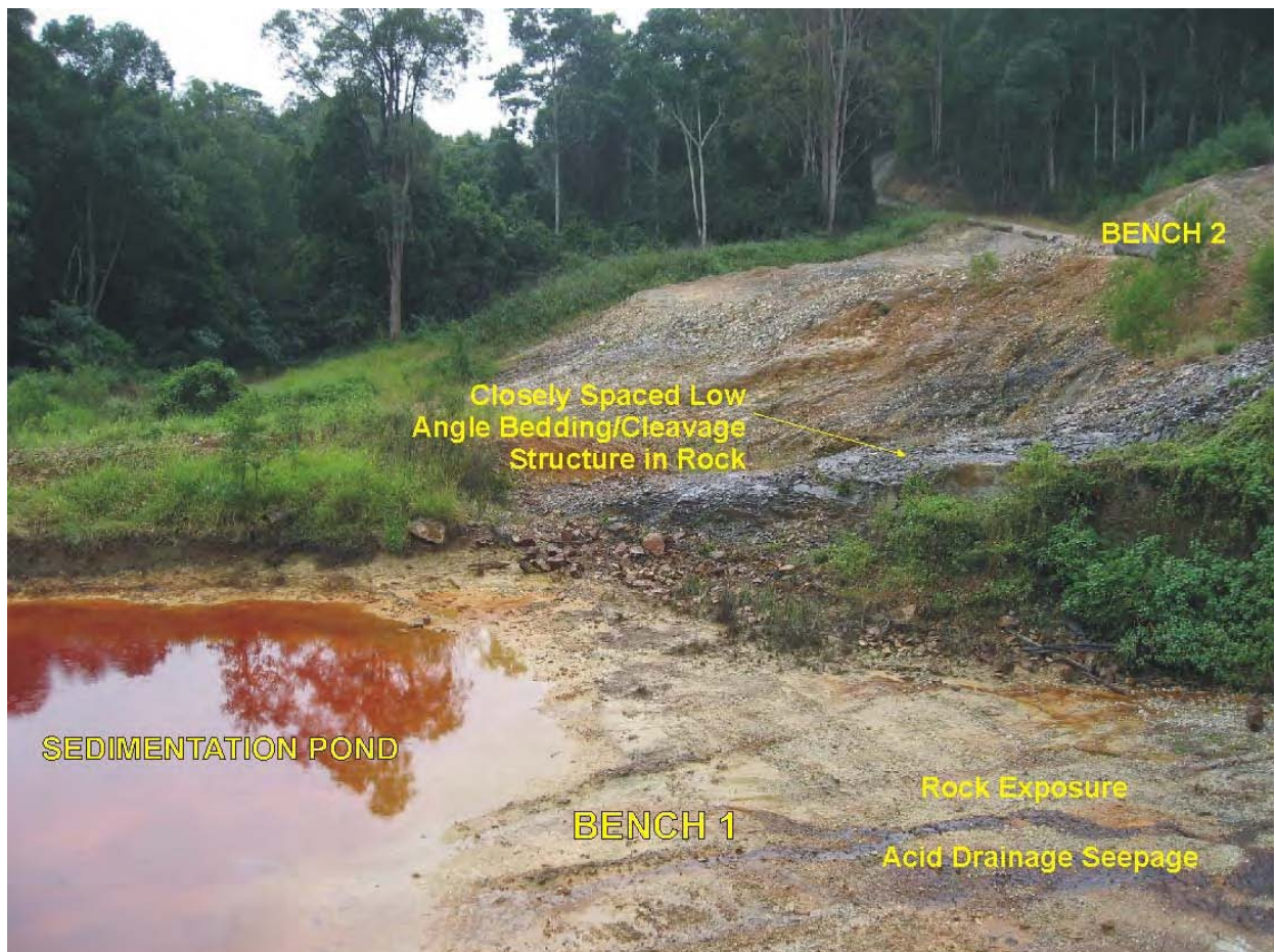
Bench 1 Acid Drainage Seepage Exposure (Photo 8113 – 18/5/09)
