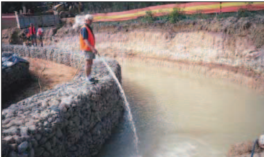
Figure E2. Poor gypsum application technique.
