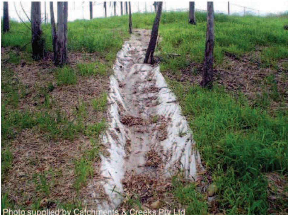
Clean water diversion drain or chute
