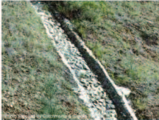
Photo 1 – Permanent, grouted-stone batter chute
