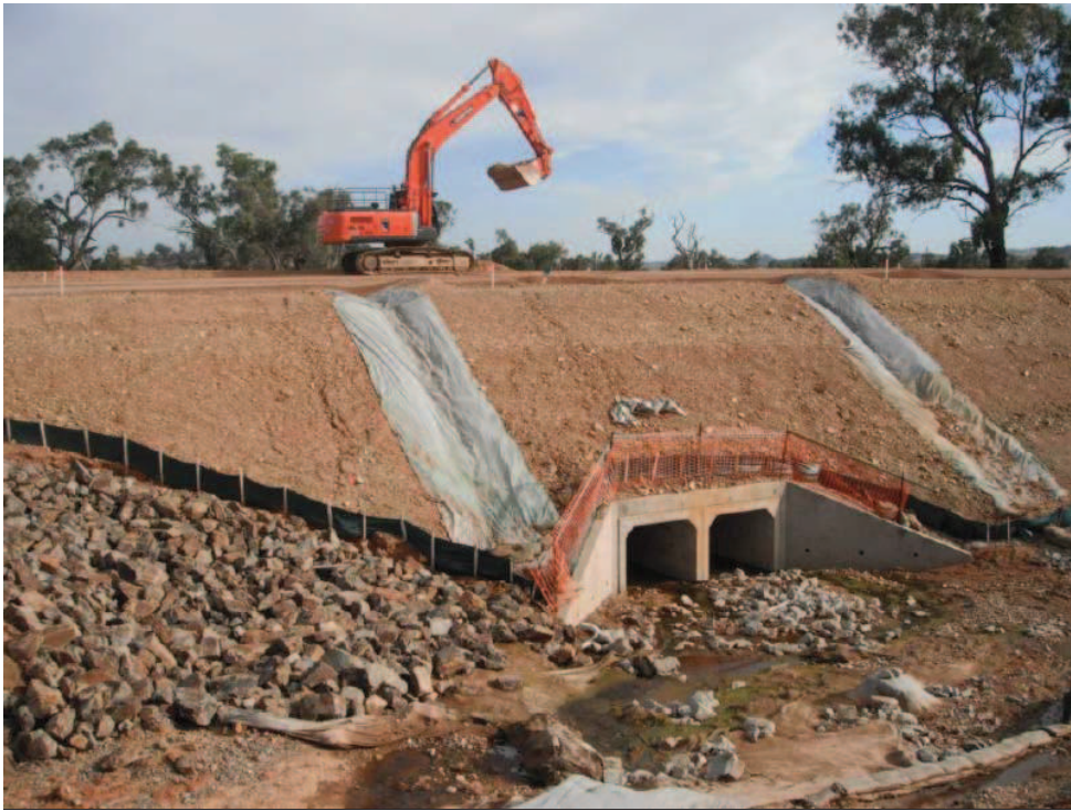
Temporary Batter chute
