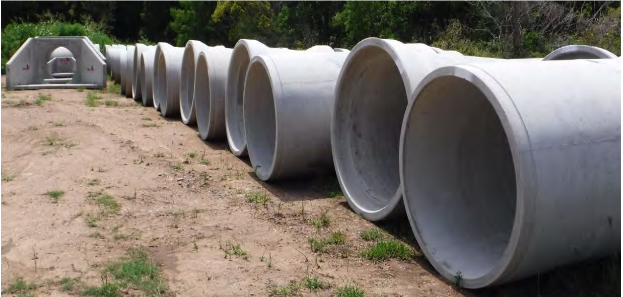
Figure 3 – Stormwater drainage on site ready for installation.
