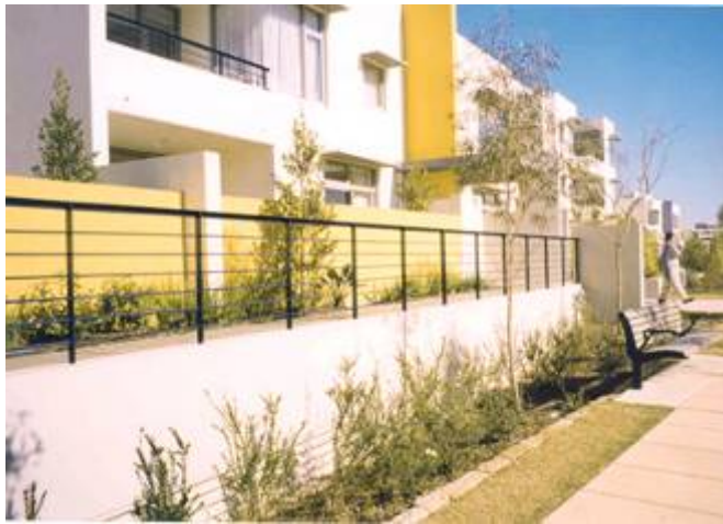
Example of an appropriate “sub-basement” option which has been designed as an integral component of the way the building presents a transition to the public domain
