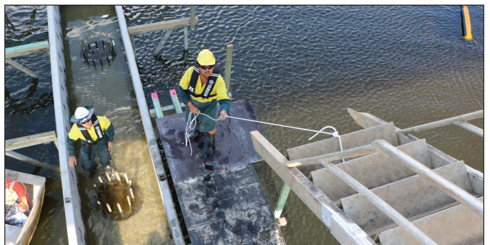
ABOVE: Tom Yeo and Nathan Warlosz lower the access steps to a work platform in the Cudgen Creek channel as Council takes possession of the site, to start construction of the bridge above the water level. The tub, now in place, will allow workers a dry workplace to begin construction of the pile cap. A working deck will be built around the tub for ease of construction.
