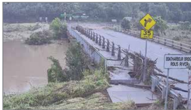
Boatharbour Bridge over the Rous River through the camera after the river subsided in March 2022.
