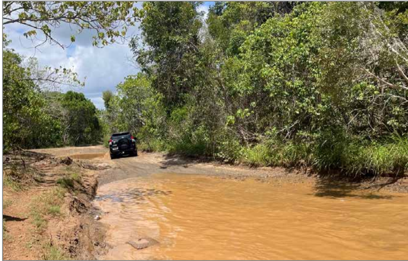
The Dreamtime Beach access track at Fingal Head is closed to vehicles and pedestrian during upgrade works.
