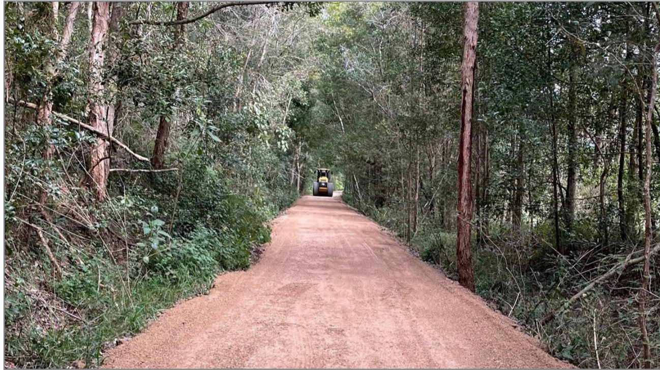
Workers making good progress last week laying down the gravel surface a few kilometres south of Murwillumbah.
