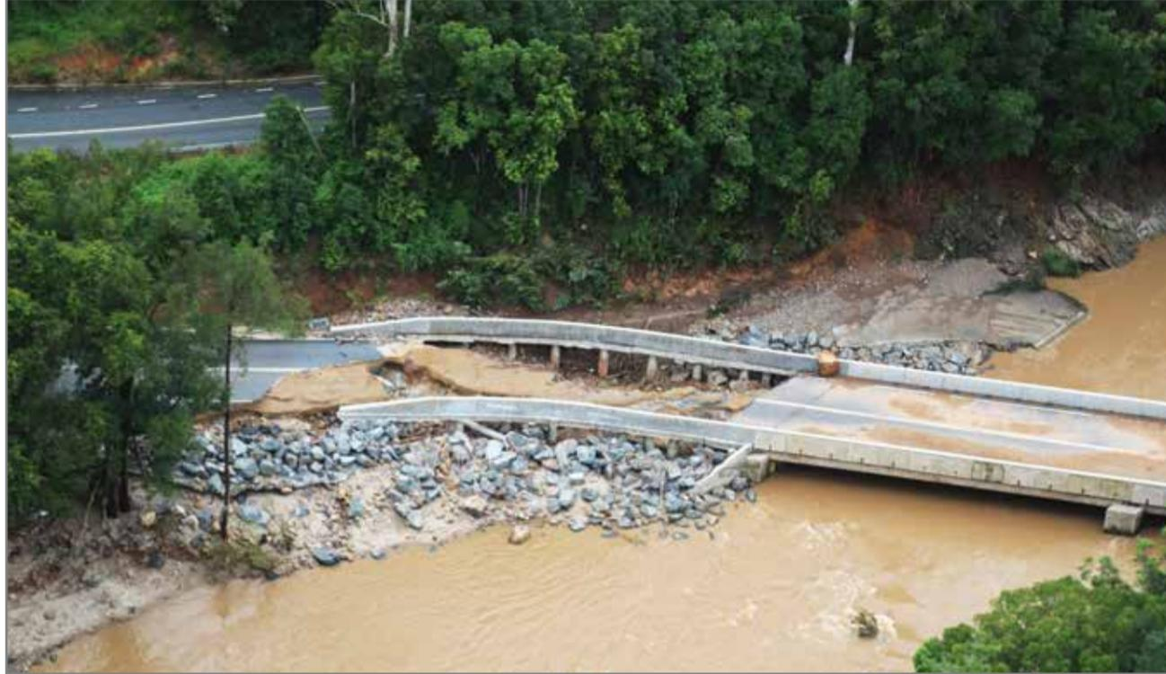
Byrrill Creek Bridge suffered severe damage in the first flood and even more during the latest deluge.
