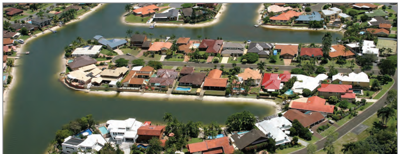
Council manages nine canal estates – comprised of both navigable and non-navigable waterways – and the foreshores adjacent to several hundred residential properties.
