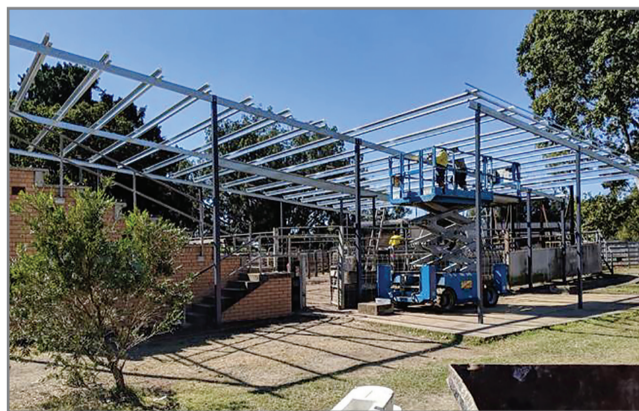
Construction of a new roof at Murwillumbah's Cattle Saleyards is part of recent improvements to community infrastructure in Murwillumbah to support economic growth.
