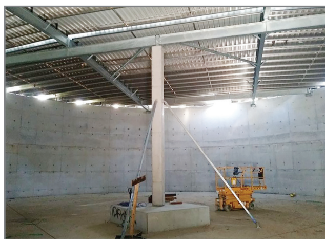
Top: The Chambers Lookout reservoir at Banora Point taking shape and (bottom) the finished product on the inside.
