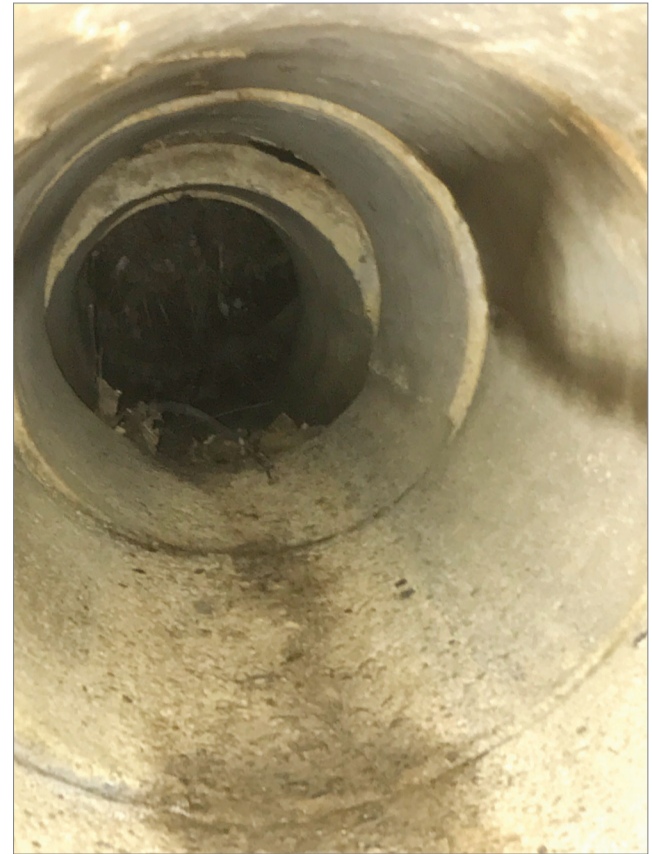
An internal view of the of the concrete pipe which was displaced during the March 2017 floods.
