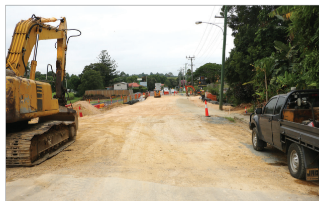
Tweed Valley Way at Blacks Drain worksite is prepared for kerb and gutter installation and then the final asphalt seal will be applied.
