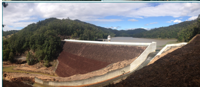
Environmental Scientist Greg Lollback bird watching at the dam wall (top left). The nest of a Speckled Monarch (top right). The wall of the dam will be raised 8.5 metres (bottom).
