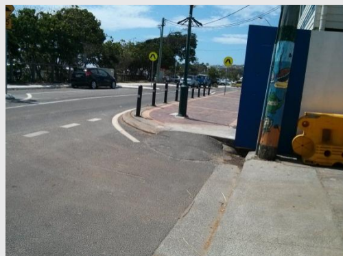
Poor temporary kerb ramp at Marine Parade
