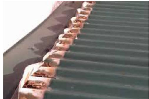
*Colorbond roof galvanic corrosion caused by lead flashing*
