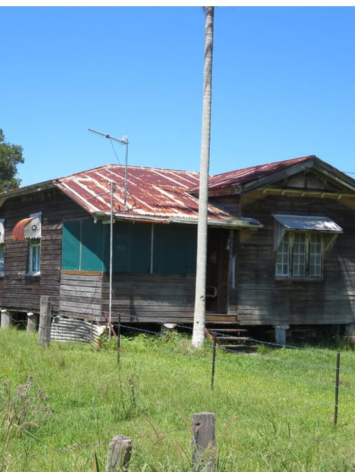
*Patterns of rusting on old galvanised steel roof and window hoods. Replacing these roofs should be with like materials and sizes as modern materials alter the appearance and can lead to chemical reactions between materials.*
