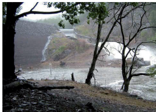
Spillway January 2008 during minor flood.
