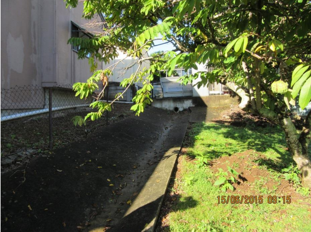
Point of discharge No. 764 Terranora Road approximately 15m from shared boundary
