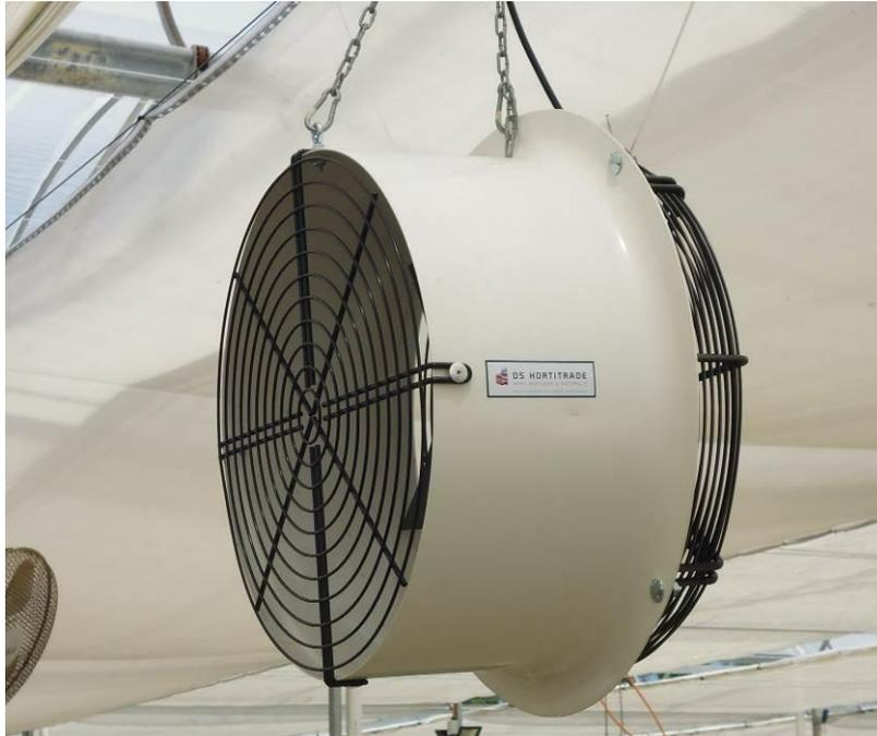
**Photograph 1:** HAF fans installed in the facility
